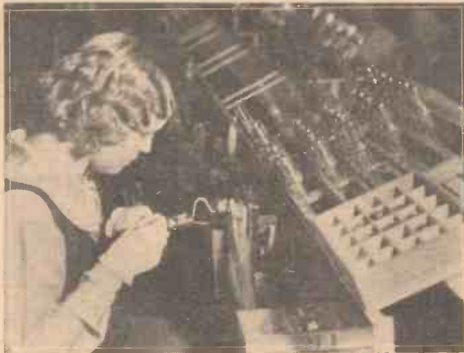
A spot-welding machine in use at the Cossor Works at Highbury.
