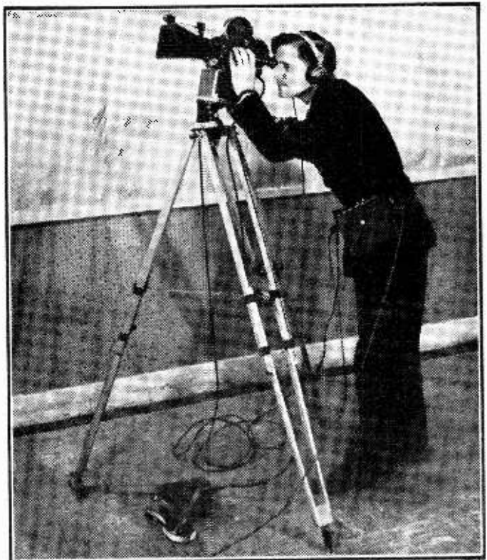
The lightweight camera referred to on the left, with a magnetic recorder between camera and tripod head. The mike amplifier, slung from the operator's waist, is transistorised.
