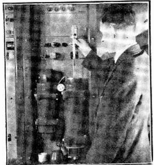
The output stage of a Marconi HM 200 U.H.F. F.M. Radio Terminal.
