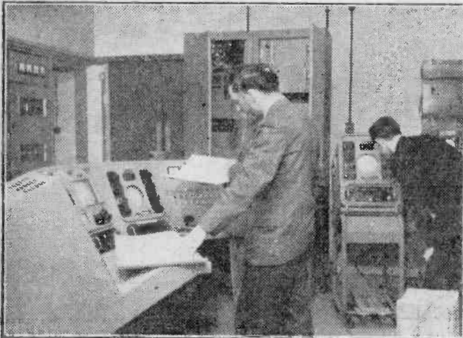
First photographs of the new Marconi medium-power Television installation at Kirk o'Shotts. These illustrations show the control desk and part of the 5 kW. transmitters with Marconi and BBC engineers during preliminary tests.
