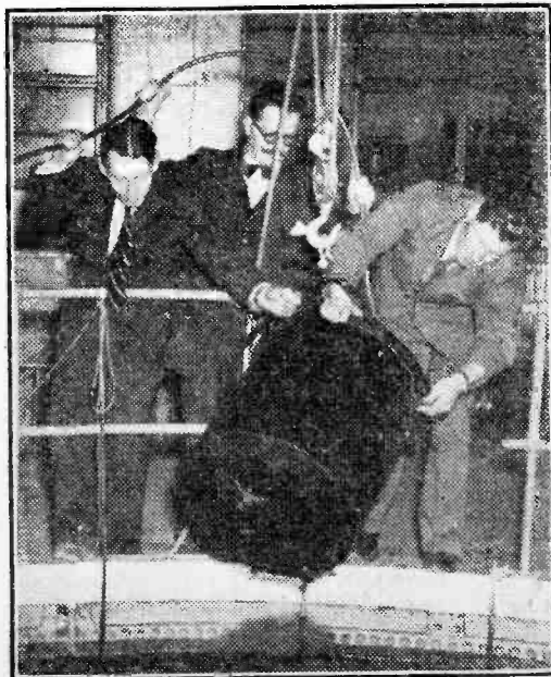
Engineers preparing to lower the underwater TV camera in its pressure casing, into the test tank.
