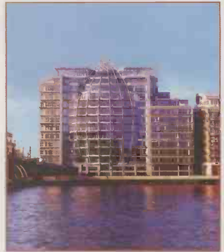
Ofcom's Riverside House HQ
