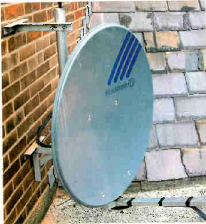
Figs. 12 and 13: 65cm Hirschmann dishes fixed on T & K wall brackets.
