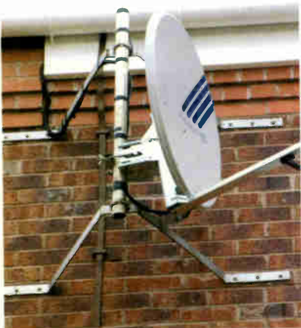
Fig. 14: A 75cm Hirschmann dish fixed on a pair of 600mm tripod stand-off brackets.
