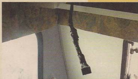
Make cables into a tidy loom with PVC tape.
