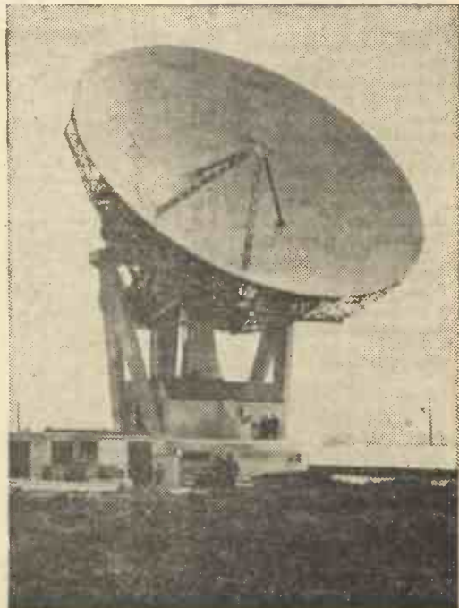
Goonhilly Downs Receiving Station.
