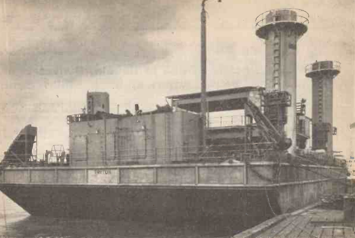
A view of "Triton" as construction nears completion.
