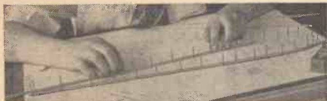
Fig. 1.—Positioning the fuselage outside strips.
