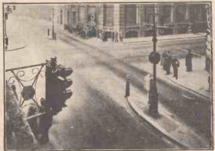
Fig. 2.—The first vehicle-actuated signal erected at the junction of Cornhill and Bishopsgate. The small crowd gathered to watch it in operation. Installation in 1932 was by Automatic Telephone and Electric Co., Ltd.
