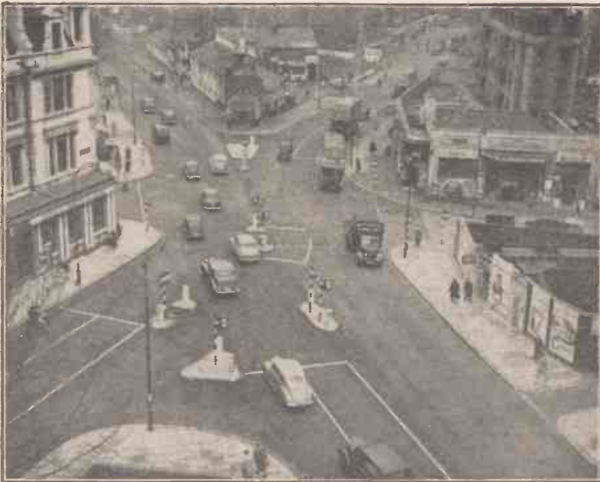
Fig. 5.—A junction of six roads at Swiss Cottage, Hampstead, where an Autoflex installation smoothly handles heavy traffic.
