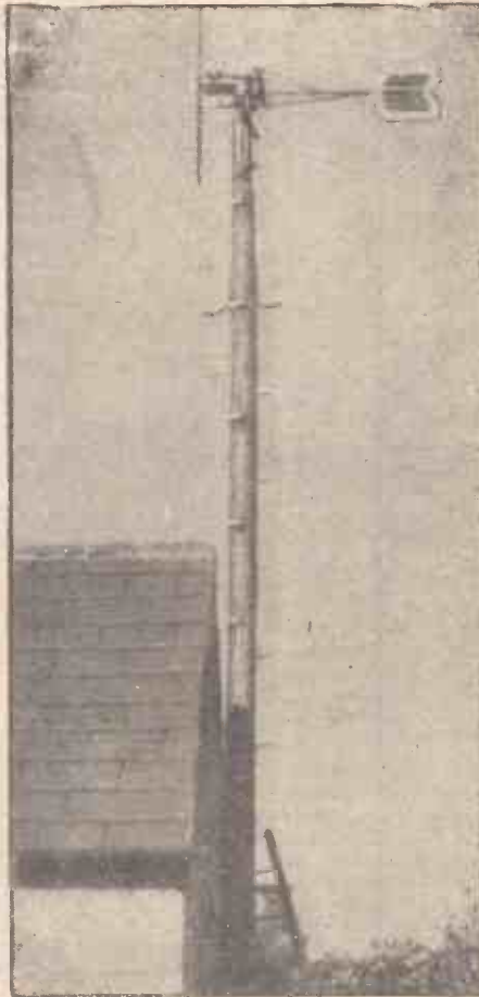
View of a complete plant. The small blocks seen along the front of the pole carry the copper conductors. One row of climbing steps can be seen on the right of the pole.
