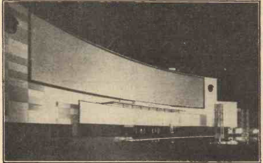
Screen with an area of 600 square metres (60 metres wide and 10 metres high) at the Palace of Light at the Universal Exhibition of Paris, 1937, on which was shown the film "Au fil de l'Eau" projected with Professor Chrétien's Hypergonar at the request of the Compagnie Parisienne de Distribution d'Electricite.
