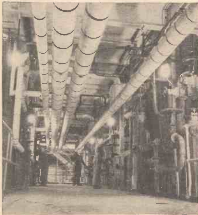
Penicillin fermenters of 5,000 gallons capacity, as used in the Glaxo Laboratories.
