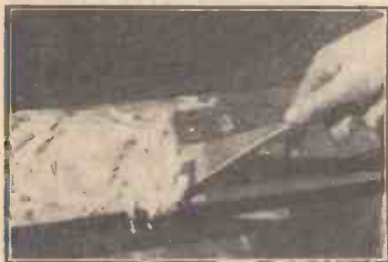
A thick film of softened and disintegrated paint being scraped away after treatment with a paint remover.
