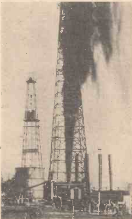
A gusher liberating black oil in a pressure stream into the air.
