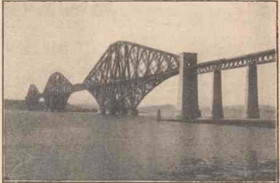
Fig. 6.—The Forth bridge—Sir Wm. Arrol & Co.
