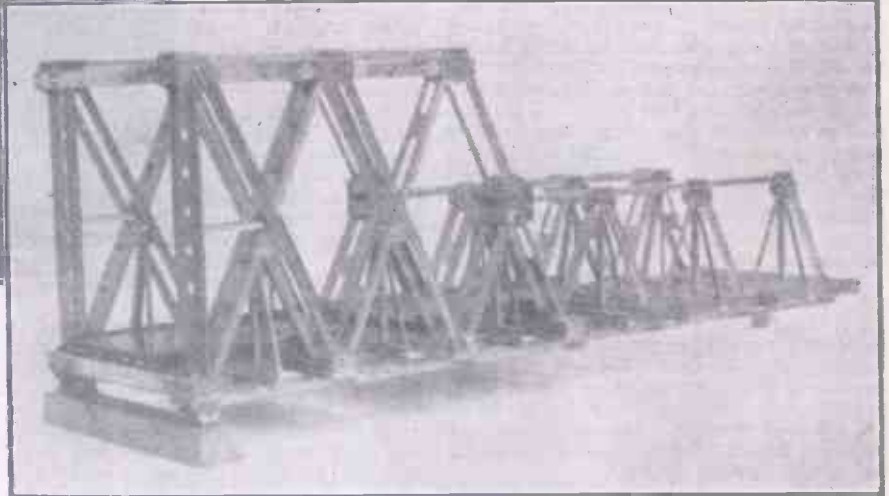
Fig. 6.—Model of the Callender-Hamilton Unit Construction Bridging made by Mr. B. E. Timmins.
