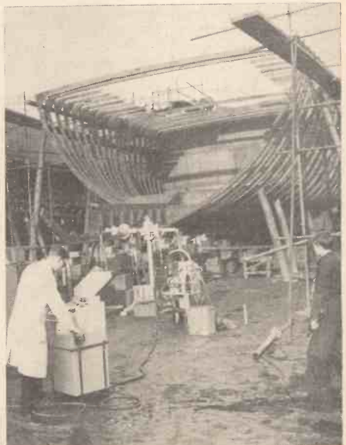
Portable X-Ray equipment is being used in a Clydeside shipyard for finding faults in electric welding. The illustration shows a welded keel in the shipyard being photographed by the X-Ray unit.
