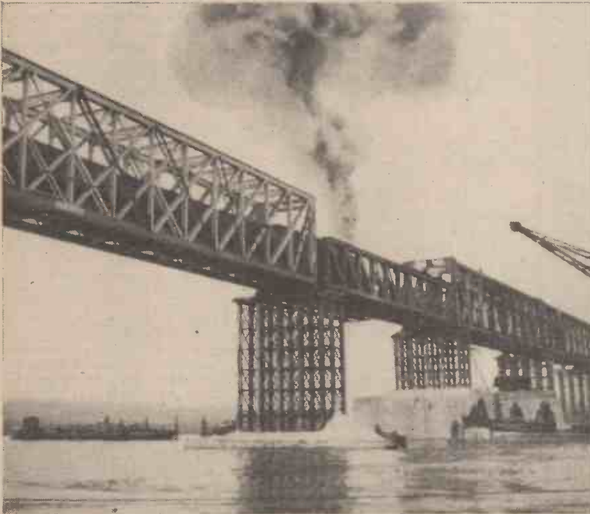
Only half a year after the total destruction of the Oosterbeek railway bridge, near Arnhem, the first train passed over the emergency bridge.
