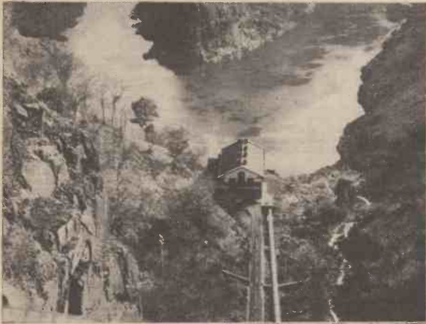
Fig. 1.—Victoria Falls power station. The lower portion of the track is seen beside the pipeline.
