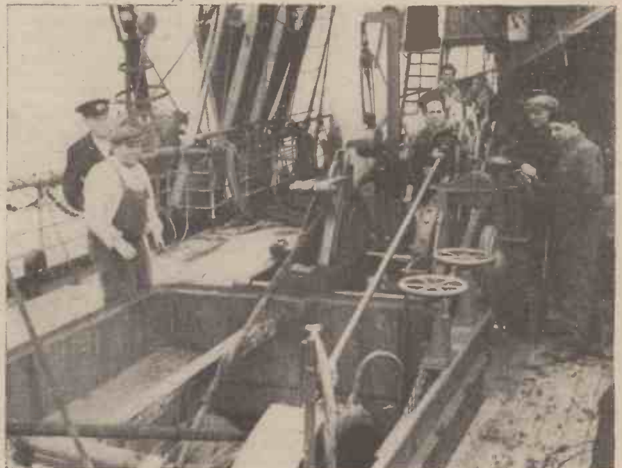
This illustration, taken on board the Great Northern Telegraph Company's cable ship "Edouard Swenson" illustrates part of the work of repairing a fault in the cable between Newbiggin, Northumberland, and Marstrand, Sweden. In the illustration the cable is seen being brought in by the cable engine to go into the cable tank.
