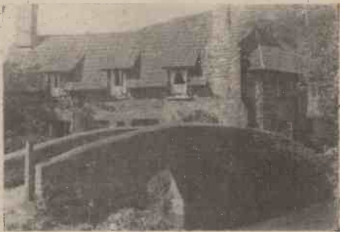
Allerford Packhorse Bridge, Somerset.
