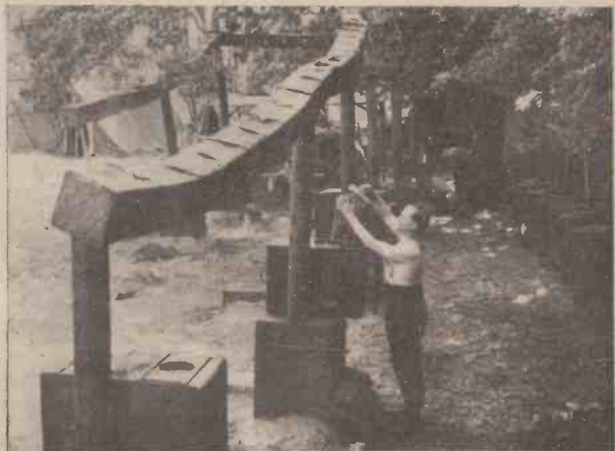
R.A.F. cooks of the 2nd Tactical Air Force improvised a first class kitchen with disused petrol cans and oil drums. An ingenious chimney of petrol cans takes the smoke from the field kitchen into the nearby trees.
