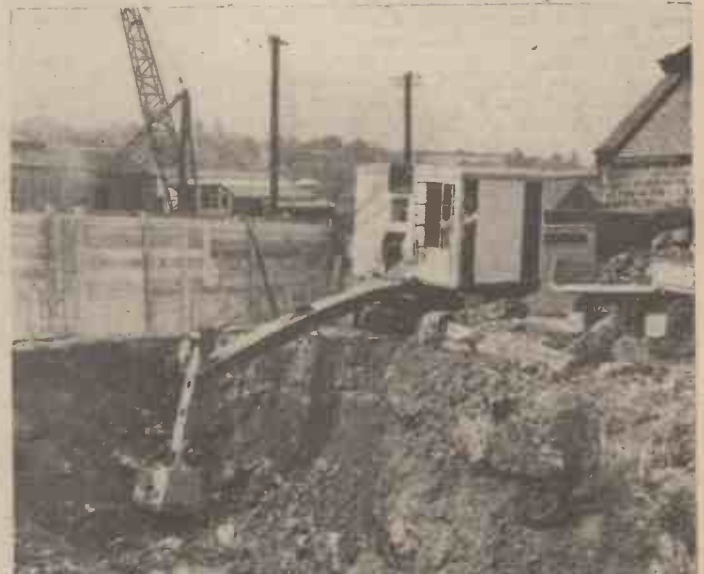
Fig. 3.—A \frac{1}{2} yd. excavator (trencher) digging for building foundations.
