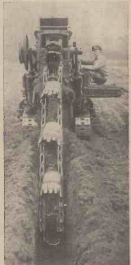
Fig. 6.—A trench-digging machine used by the Canadian Army in this country. It can dig a trench 5ft. deep and 500yds. long in one day, and is operated by one man.
