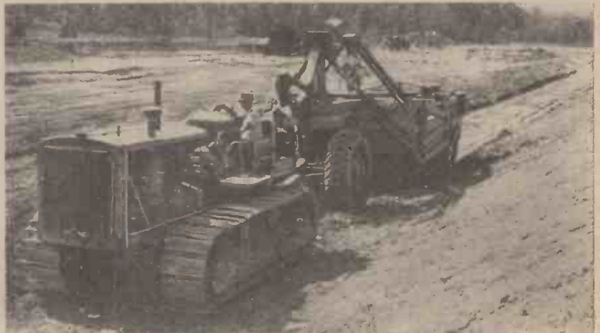
Fig. 8.—A scraper towed by a "caterpillar" diesel tractor.
