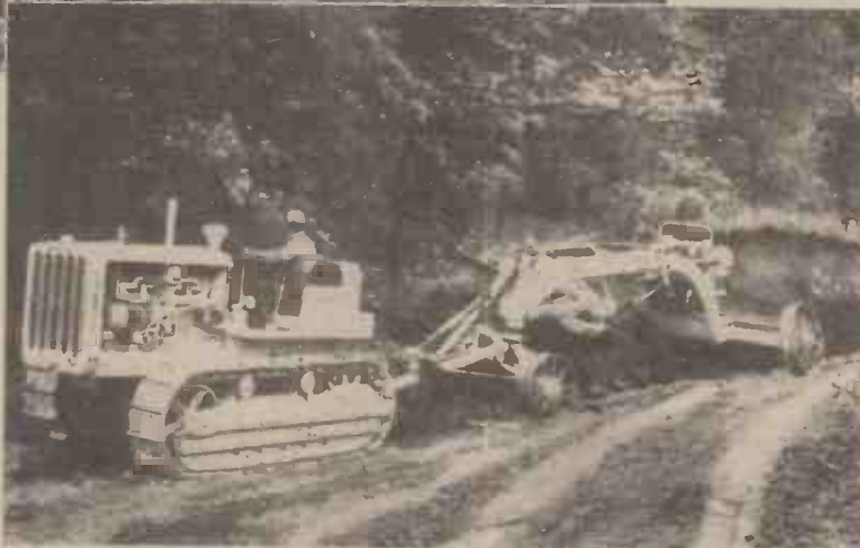
Fig. 9.—A grader towed by a diesel-driven "caterpillar."
