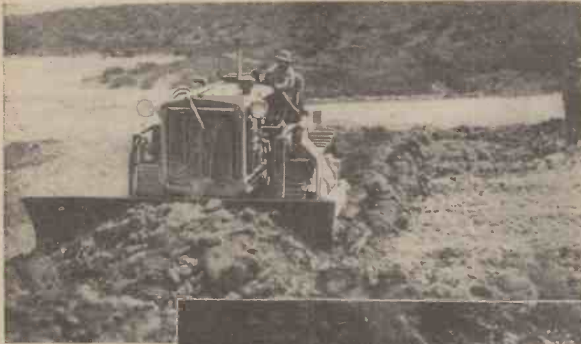
Fig. 7.—A bulldozer (American "caterpillar") at work.
