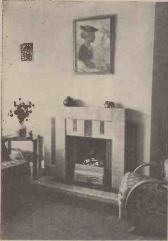
Fig. 1.—The Fulham grate in a sitting room.
