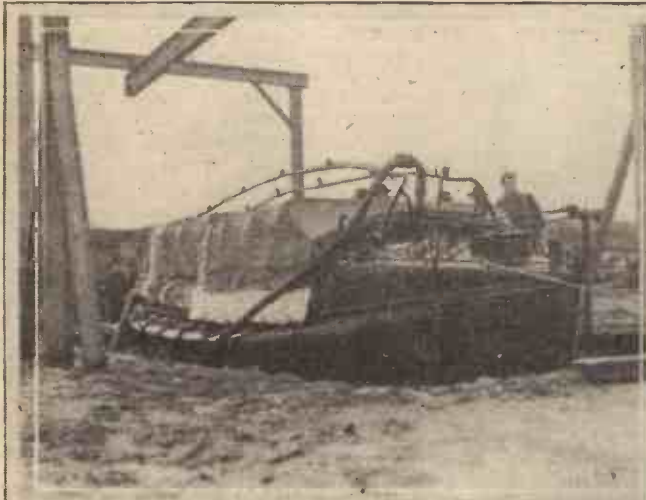
Lifeboat moored in the middle of a static water tank.
