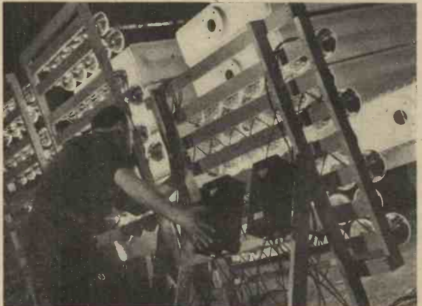
Invisible infra-red radiation is enlisted to speed up manufacture of large electric transformers at the Westinghouse plant in Pennsylvania, to help expansion of power facilities for national defence. This battery of 129 infra-red lamps cuts the paint drying time for parts of large transformers from 70 hours to 50 minutes. They have a combined energy of 32,250 watts. Development of the infra-red lamps was recently announced by Westinghouse. The 250-watt units combine lamp and reflector in a single hermetically-sealed lamp. They produce a narrow, concentrated beam of radiant heat energy, with less than 5 per cent. of total energy emitted as visible light.
