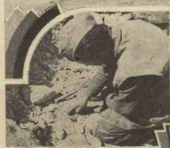
Much of the desert is rocky, and explosives have to be used before the guns can be safely placed. The illustration (left) shows a sapper placing ammonia in a hole for blasting purposes.
