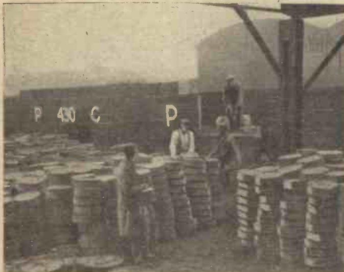
The finished product. Asphalt blocks being loaded into railway waggons for quick despatch to factory and other building sites.
