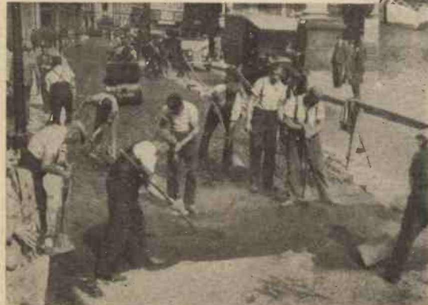
The making of an asphalt road. In the foreground, natural rock asphalt powder is being scattered on the road "bed." The illustration shows the asphalt being raked and tamped into position, whilst in the background is seen the mechanical rolling of bitumen-coated granite chippings on the asphalt surface in order to provide a non-slip surface.
