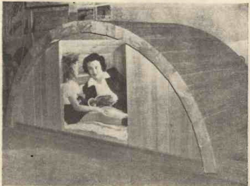
Exhibited at the New York 1942 Inventors' Exposition. A solid timber portable air-raid shelter in which three people can sleep in safety. It can be set up in 10 minutes, and no metal or nails are used.
