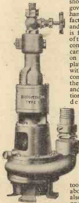
Fig. 2.—A "Broomwade" pneumatic trench pump.
