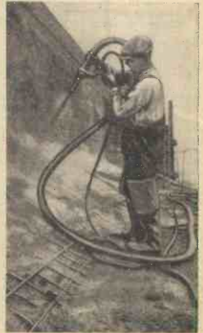
Fig. 2.—"Gunitite" being applied to a harbour wall. Note the steel reinforcement.
