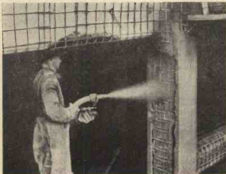
Fig. 5.—A nozzleman shooting "Gunite" for reconditioning pier supports.
