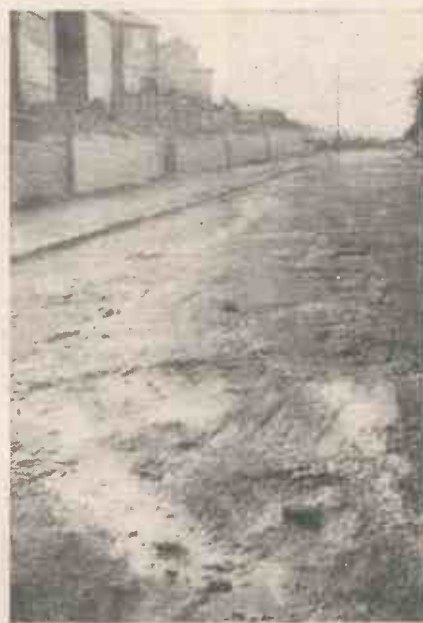
A good example of the action of rain in washing away soil, and lighter stones, is to be seen in the case of any newly made road before paving, particularly after a heavy rainstorm.
