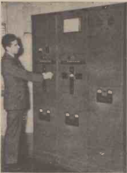
Fig. 4.—The first two panels (from the left) mount amplifiers, channels 1 and 2 respectively; on the right-hand panel are monitory loudspeakers and the announcer's emergency amplifier.
