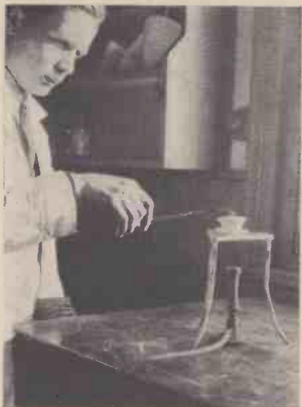
Left.—Making boric trioxide by fusing boric (boracic) acid in a crucible
