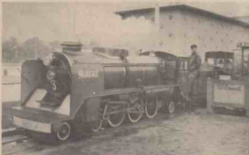
A 4-6-2 24-in. gauge locomotive
