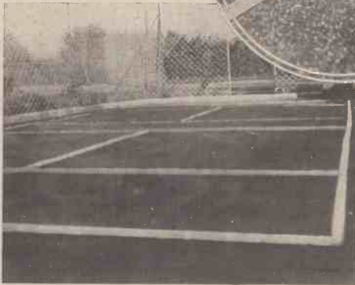
(Left) The completed court.
