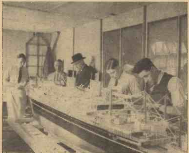
Putting the finishing touches to a 16 ft. long model of the "Dominion Monarch."
