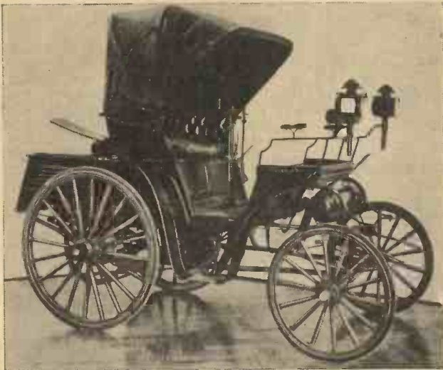
The first hooded car, the Daimler model of 1894. Its design marked an important advance in commercial car construction.
