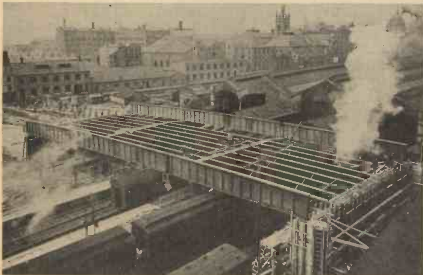
The new bridge under construction at Durham Street, Belfast
