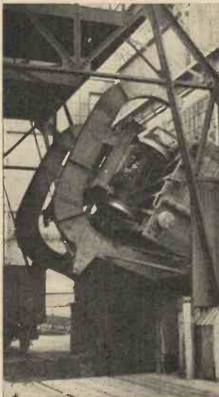
The mechanical acrobat which automatically feeds coal to furnaces.
