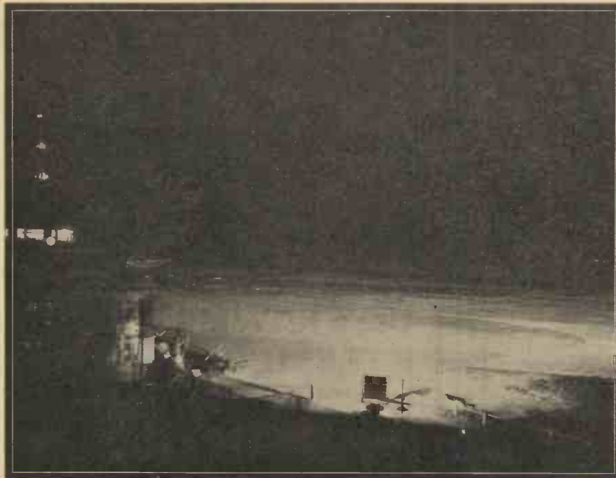
The London air-port, Croydon, floodlit at night.
