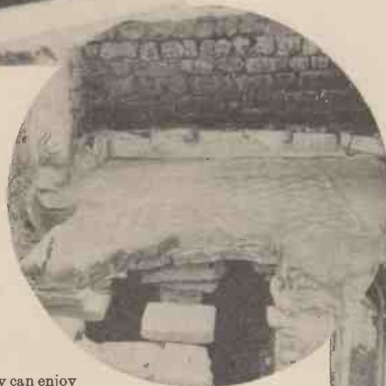
Central heating 2,000 years ago. A room in a Roman villa at Chedworth; note the mosaic floor and flue beneath for heating.
