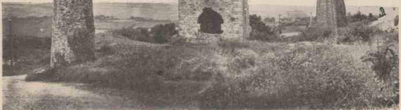
The ruined engine house of a 300-year-old Cornish tin mine. It was in ancient tin mines such as this that Savery's engines were applied.
