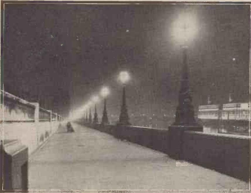
A night scene on the Albert Embankment. The main thoroughfare is illuminated by 400-watt lamps, while the "Dolphin" standards which stud the whole length of the parapet have been adapted to accommodate 250-watt "Osira" lamps.
