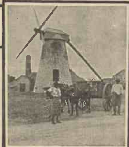
(Above) A tower mill which is hand operated for changes in the wind, at Barbados. The sails are moved round by a long pole. As the trade winds in Barbados blow steadily in the same direction for nine months in the year, it has not been necessary to fit automatic gearing; and (right) a modern circular mill at work in British West Indies.
