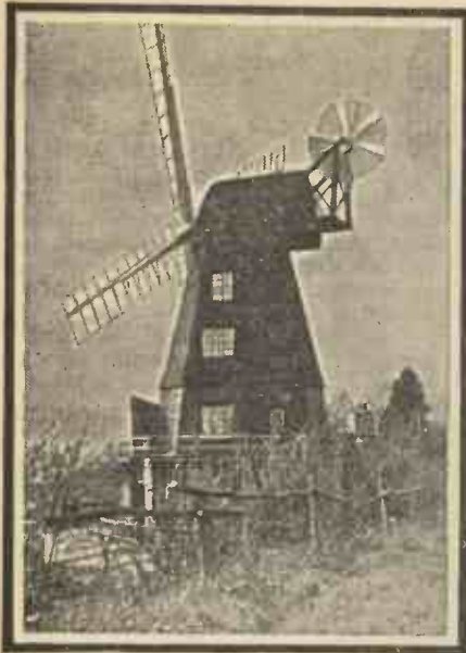
A three-quarter smock mill at West Chilington, Sussex, so called because the wooden casing goes over the mill like a smock for three-quarters of the height of the tower.
