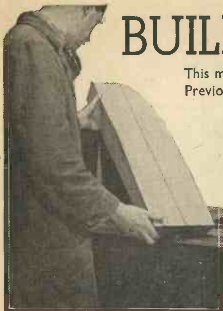
Fig. 2.—The hull in course of construction, showing imaginary chine line.
