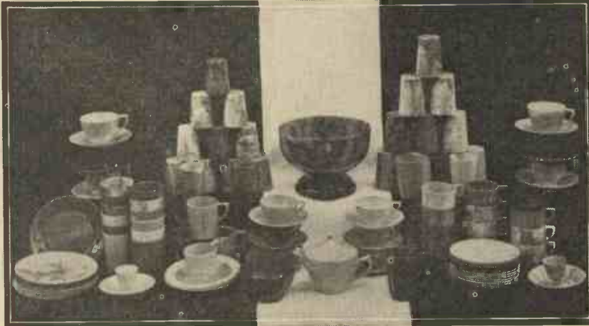
A display of unbreakable table ware, made of "Beal" urea-formaldehyde plastic.
