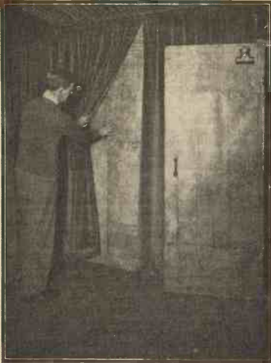
Fig. 1.—Indicating how the whole of the interior of the spot-light studio is completely lined with copper sheet to prevent radio-frequency interference.
