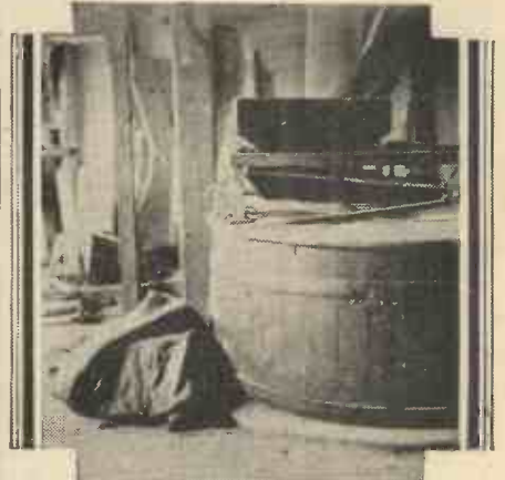
A view of the interior of a cutting mill. The stones rotate inside the wood casing.
