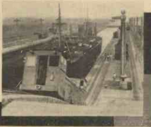
(Above) A bridge over the Welland Ship Canal, Ontario, Canada. (Right) Towing a ship through Gaton Lock. The electric loco is seen climbing to the level of the second lock (four locos are used to each vessel).
