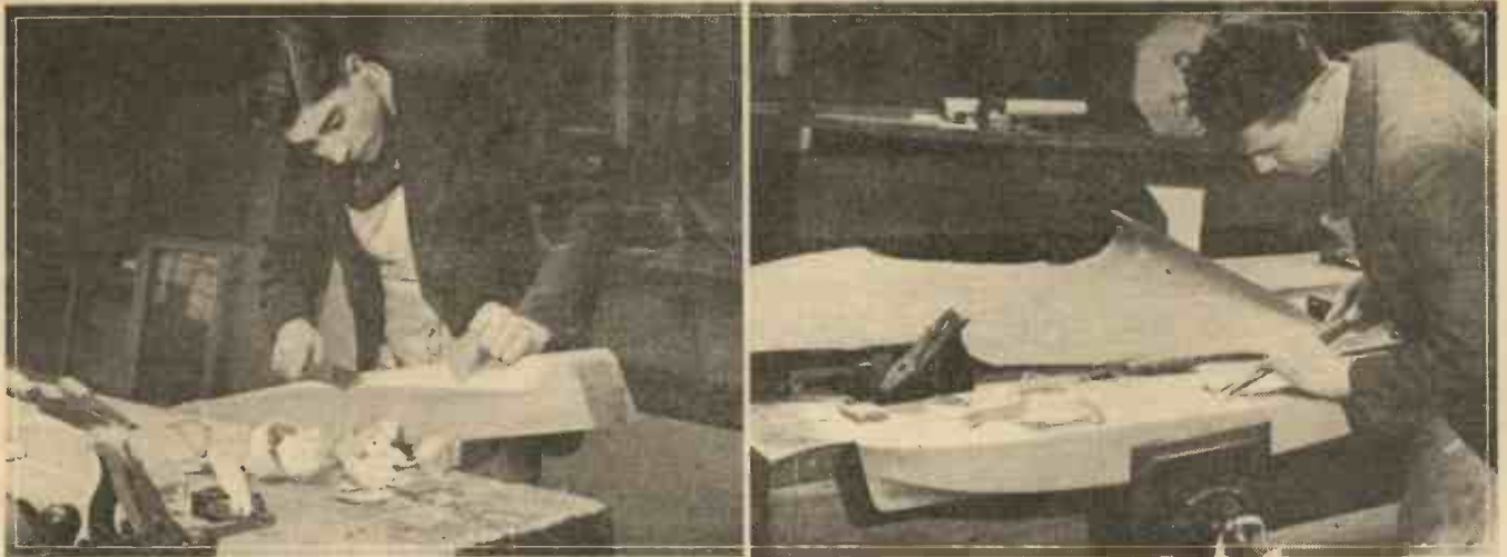
Two photographs showing constructional work on the hull in progress.
