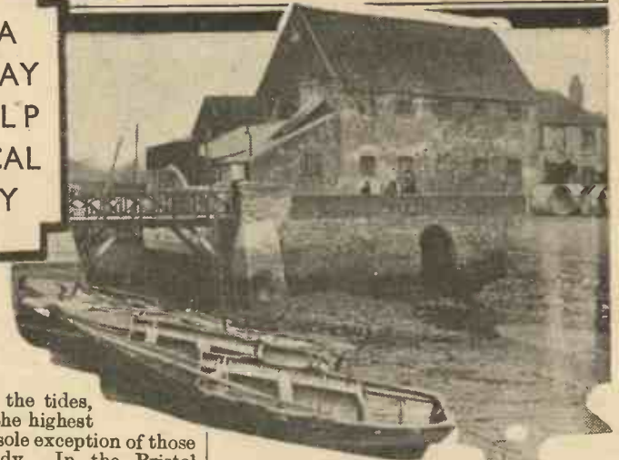
Emsworth Tide Mill from below the dam at low tide.
