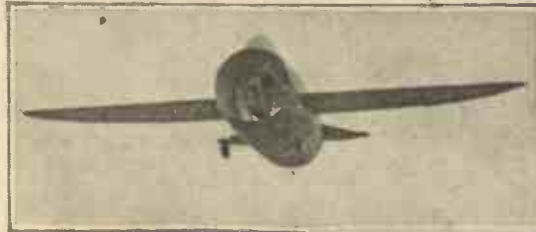
An aeroplane which employs a tubular fuselage which it is claimed has great stability and speed. The two photographs show the 'plane in the air and on the ground.
