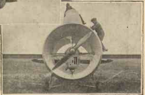
An aeroplane which employs a tubular fuselage which it is claimed has great stability and speed. The two photographs show the 'plane in the air and on the ground.
