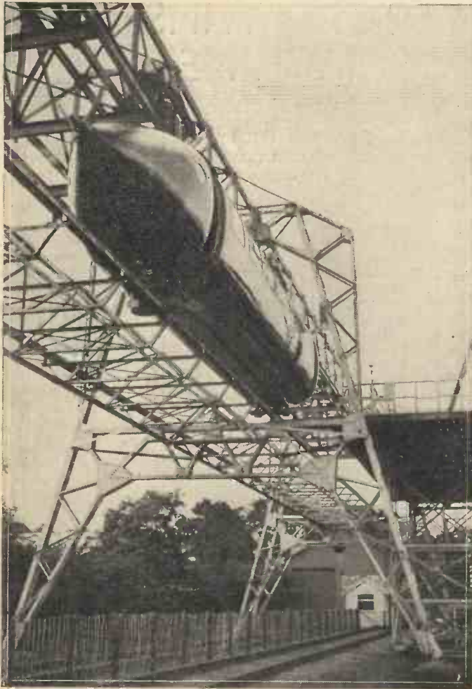
A demonstration railplane, showing the method of erecting over existing railway lines near Glasgow.
