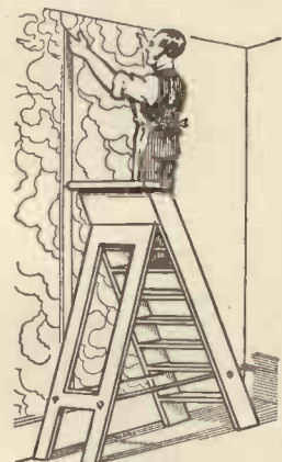
All kinds of House Decorating and Repairing can be done.
