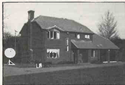
Just for interest – Thorn EMI's purpose-built experimental automated house.
