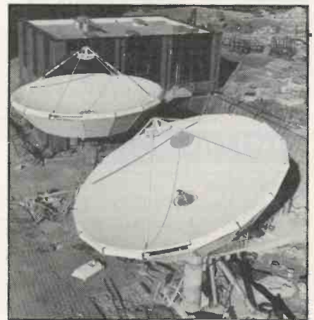
The IBA's two eight metre diameter satellite up-link dishes in preparation.
