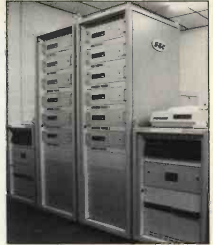
SSI cubicles and technicians terminals at Inverness signalling centre
