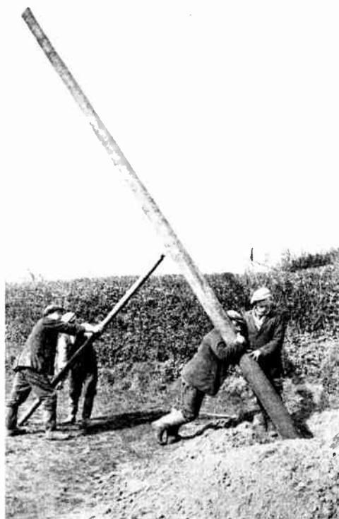
Fig. 33.—ERECTING L.T. POLE—SECOND STAGE.
