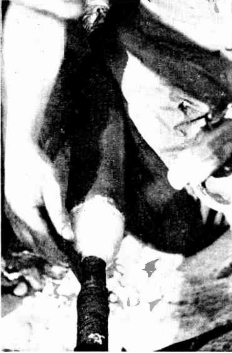
Fig. 50. L.T. STRAIGHT-THROUGH CABLE JOINT—FIFTH STAGE.
