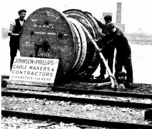
Fig. 41.—DRAWING CABLE INTO DUCT.
