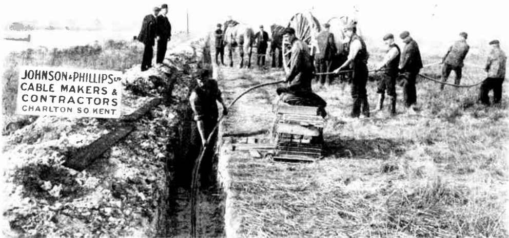
Fig. 38.—LAYING CABLE BY MEANS OF DRUM WHEELS.
