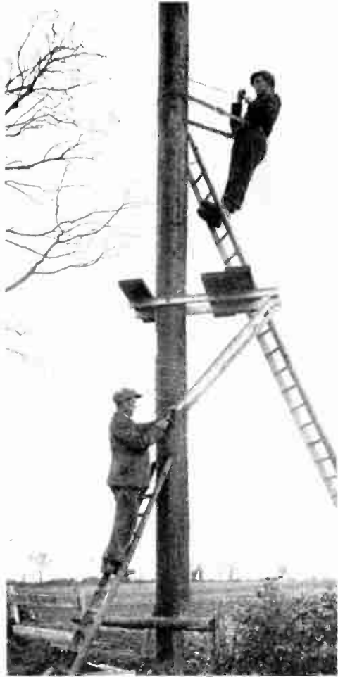
Fig. 34.—ERECTING A TRANSFORMER PLATFORM AND DRILLING HOLES FOR FIXING SWITCHGEAR.
