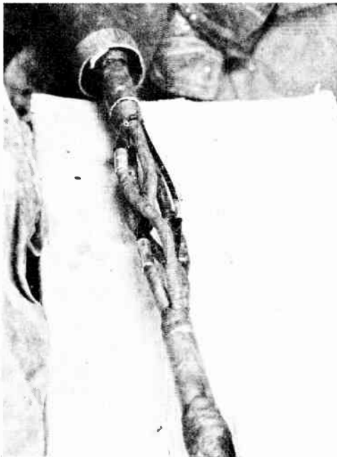
Fig. 48. L.T. STRAIGHT-THROUGH CABLE JOINT—THIRD STAGE. Showing taping of cores completed, cores cut to length and ferrules in position.
