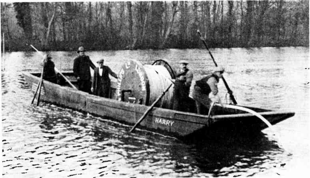
Fig. 44.—LAYING E.H.T. CABLE ACROSS THE RIVER THAMES NEAR HENLEY. ( Johnson and Phillips, Ltd. )
