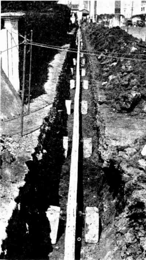
Fig. 39.—LAYING E.H.T. CABLE IN TRENCH, USING ROLLERS FOR PULLING OUT.
