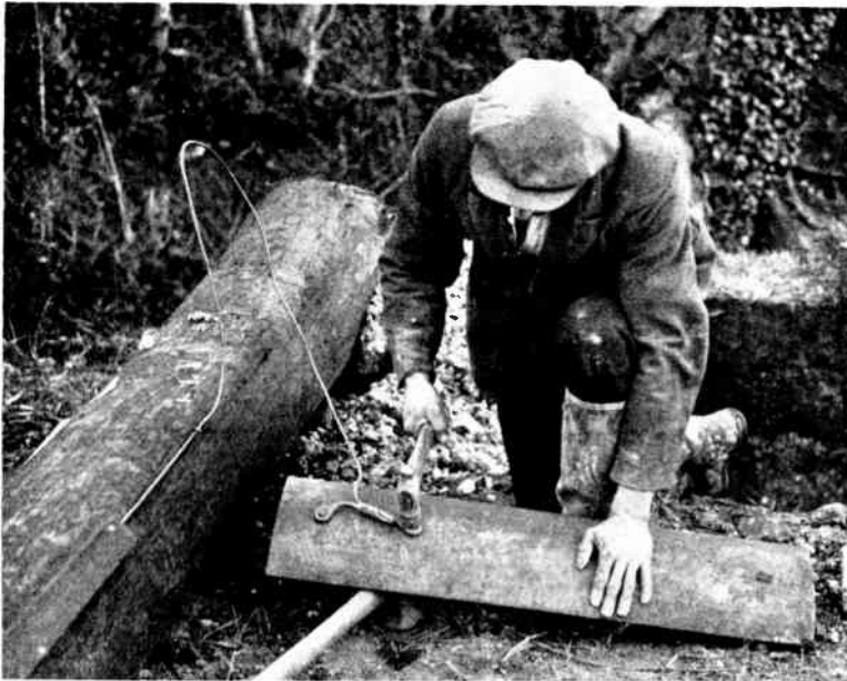
Fig. 13.—RIVETING COPPER BOND ON TO EARTHPLATE BY MEANS OF DRIFT PINS.
