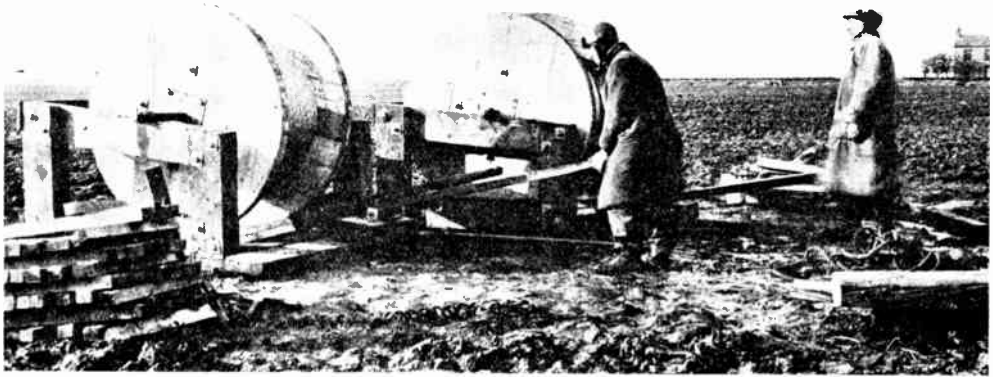
Fig. 15.—WIRE DRUMS MOUNTED ON FRAMEWORK AND CONDUCTORS BEING PULLED OUT. Note planks being used for braking to prevent drum over-running. (Johnson and Phillips, Ltd.)
