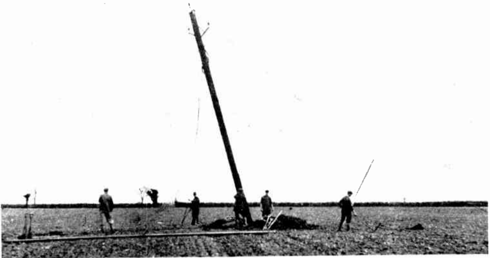
Fig. 12. —ERECTING THE E.H.T. POLE—THIRD STAGE. The pole is now almost up and the gin pole has moved along and is merely floating on the pulling rope.
