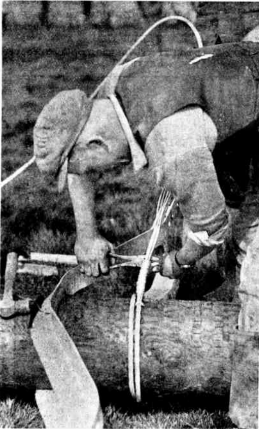
Fig. 7.—FIXING STAY WIRE ON H.T. POLE BEFORE ERECTION.
