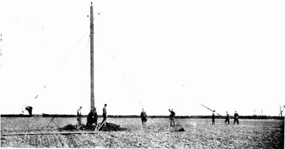
Fig. 9.—H.T. POLE IN POSITION.
