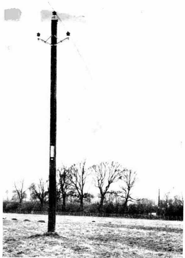
Fig. 20 --E.H.T. POLE USED ON NORWICH RURAL ELECTRICIFICATION SCHEME.
