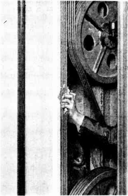
Fig. 9.—TESTING THE ROPES FOR "NEEDLES."
