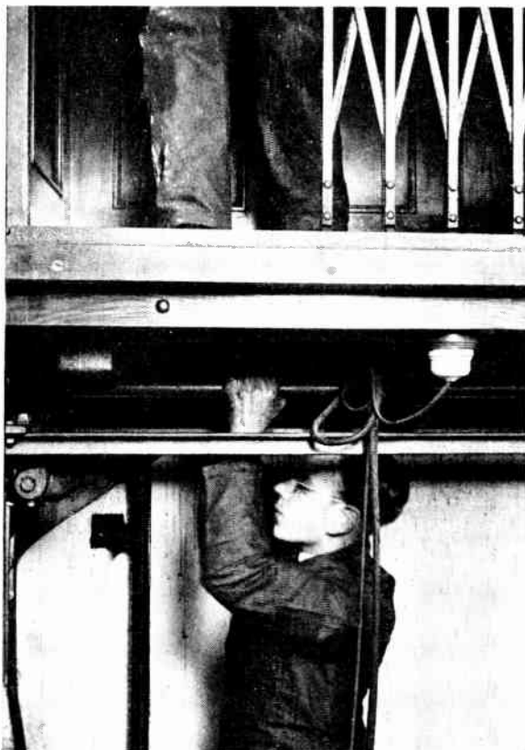
Fig. 7.— TESTING THE SAFETY GEAR.
