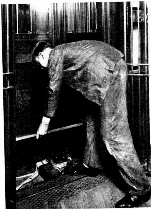
Fig. 6.—RAISING THE FALSE FLOOR OF AN AUTOMATIC PUSH-BUTTON LIFT TO INSPECT AND CLEAN THE CONTACTS.
