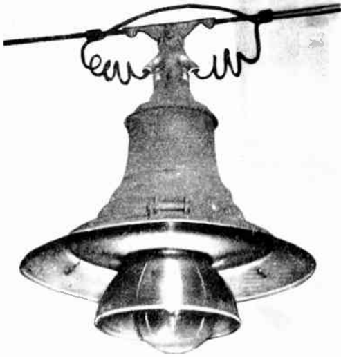
Fig. 3.—METHOD OF SUPPORTING A LANTERN FROM THE SPAN WIRES AND TERMINATING THE CABLE CONNECTIONS TO IT.
