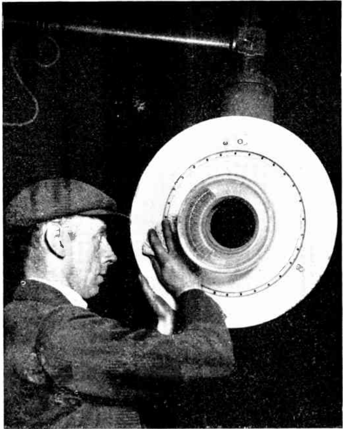
Fig. 12.—CLEANING THE REFLECTOR OF A STREET LIGHTING LANTERN.
