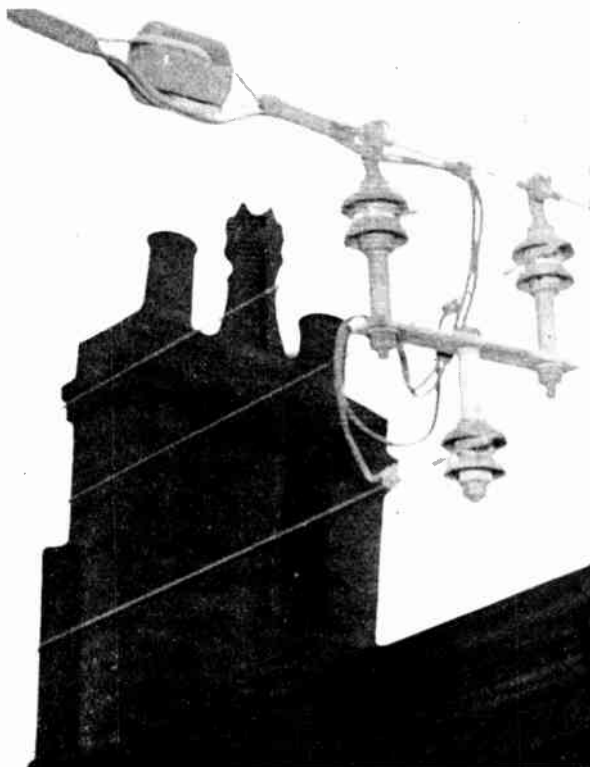
Fig. 1.—SUPPORTING THE OVERHEAD LINE BRACKETS FROM SPAN WIRES.
