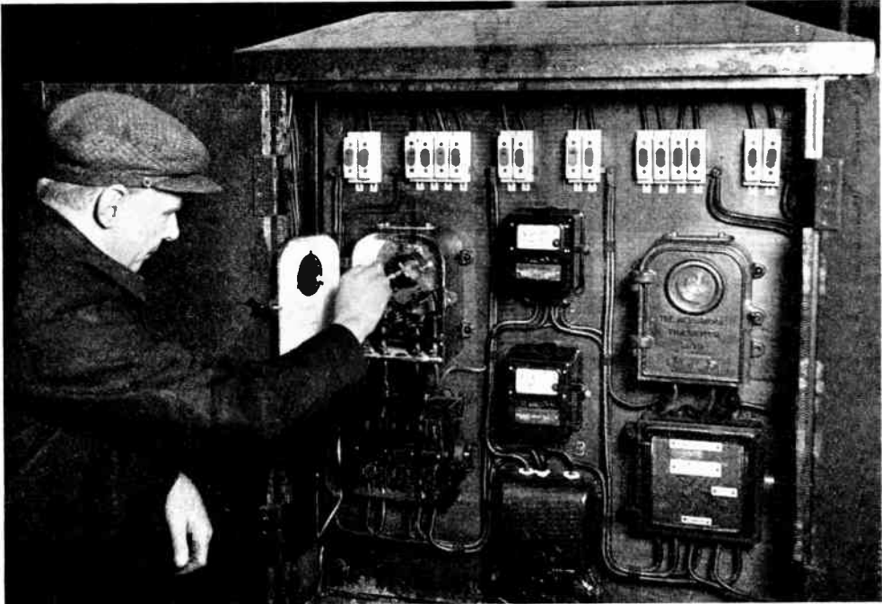
Fig. 14. —SETTING THE DIAL OF A TIME SWITCH.
