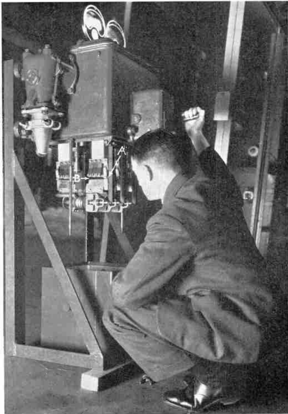
Fig. 3.—EXAMINING AN OIL CIRCUIT BREAKER TO MAKE SURE THAT THE ARCING CONTACTS (A) MAKE BEFORE AND BREAK AFTER THE MAIN CONTACTS (B). (Crompton Parkinson, Ltd.)
