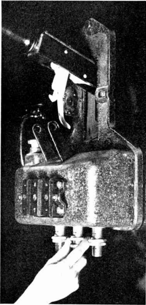
Fig. 8.—SETTING THE TRIPCOILS OF AN ORDINARY TYPE OF OIL CIRCUIT BREAKER.
