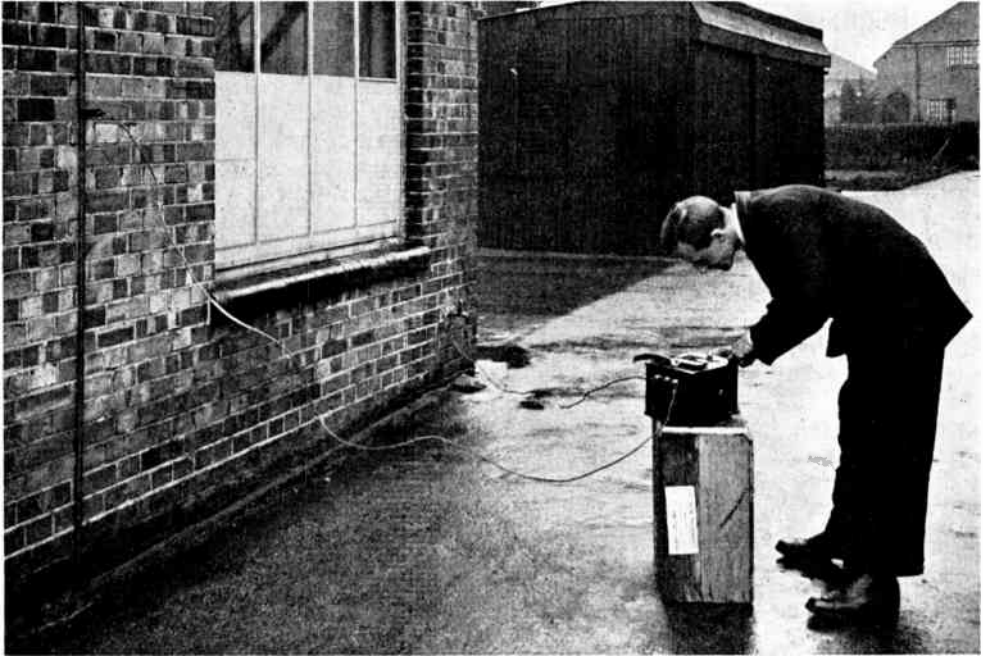
Fig. 1. —MEASURING THE RESISTANCE OF A LIGHTNING CONDUCTOR EARTH PLATE.
