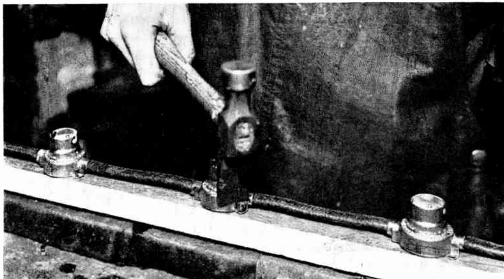
Fig. 6. —MOUNTING A BAYONET CAPPED STRIP ON WOOD BATTENS.
