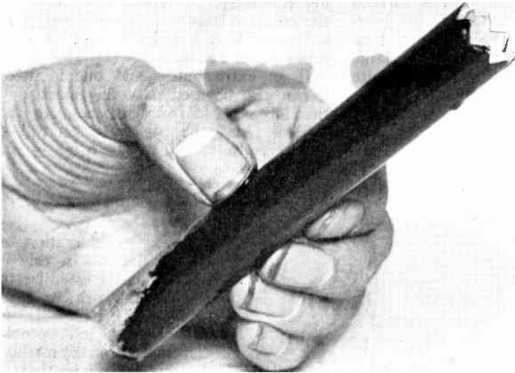
Fig. 5.—How TO CUT A HOLE IN A WALL (1).
