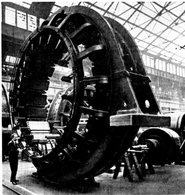
Fig. 24.—MAGNET FRAME OF 12,500 H.P. ELECTRIC WINDER.
