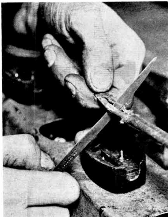
Fig. 1. —STRIPPING OFF THE CABLE INSULATION.
