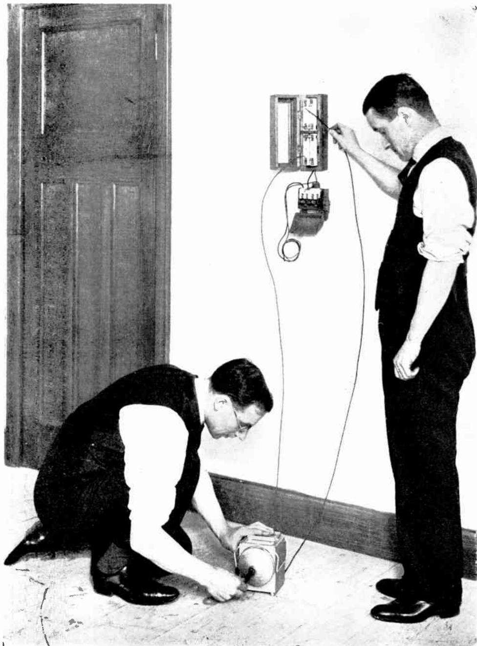
Fig. 2. —MAKING A POLE TO POLE TEST.
