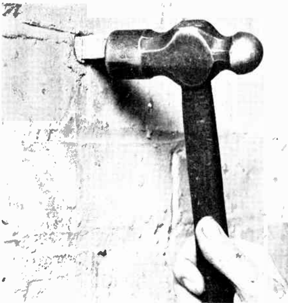
Fig. 9. —INSERTING THE WEDGE.
